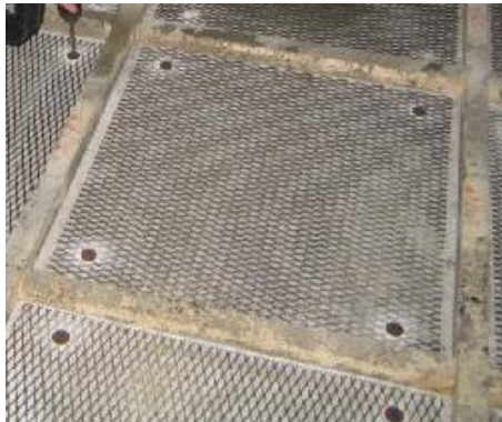
Fig. 4: Steel mesh installation
