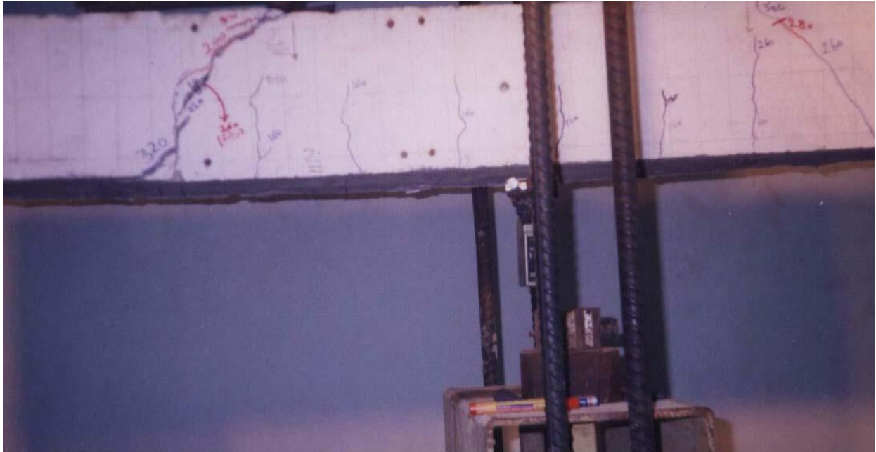
Fig. 4- Failure of Control Specimen Fcont due to Concrete Shear Failure
