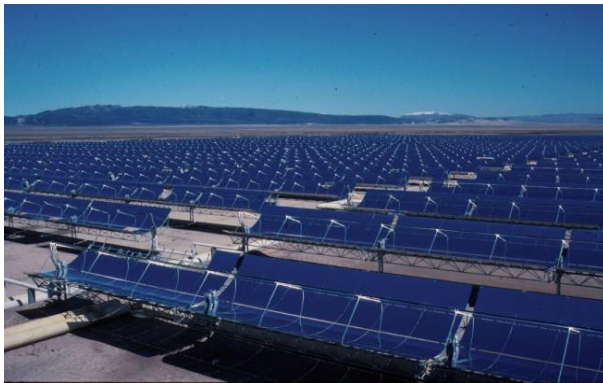
Fig. 7- Parabolic Trough CSP SYSTEM
