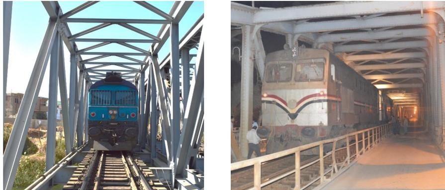
Fig. 5. Gerga & Zifta Loading Test (Locomotive Wagon)
