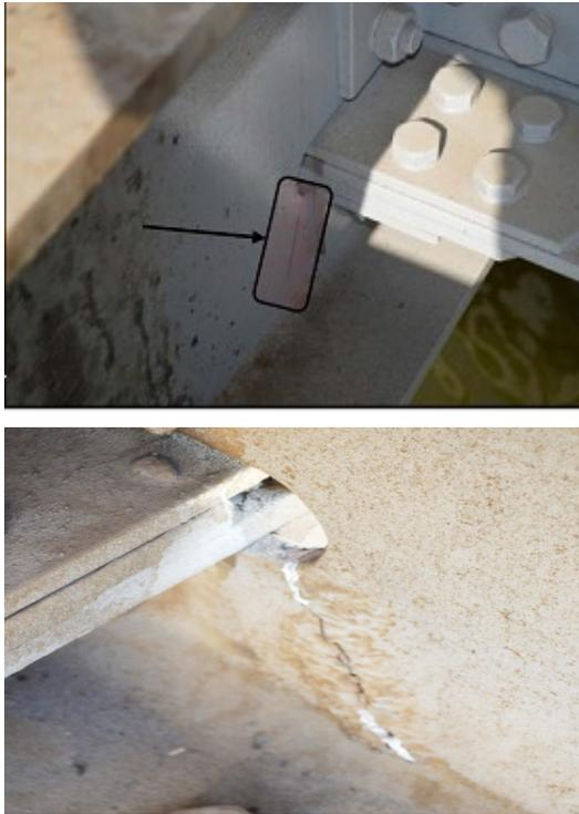
Fig. 6. Gerga railway bridge' Fatigue cracks
